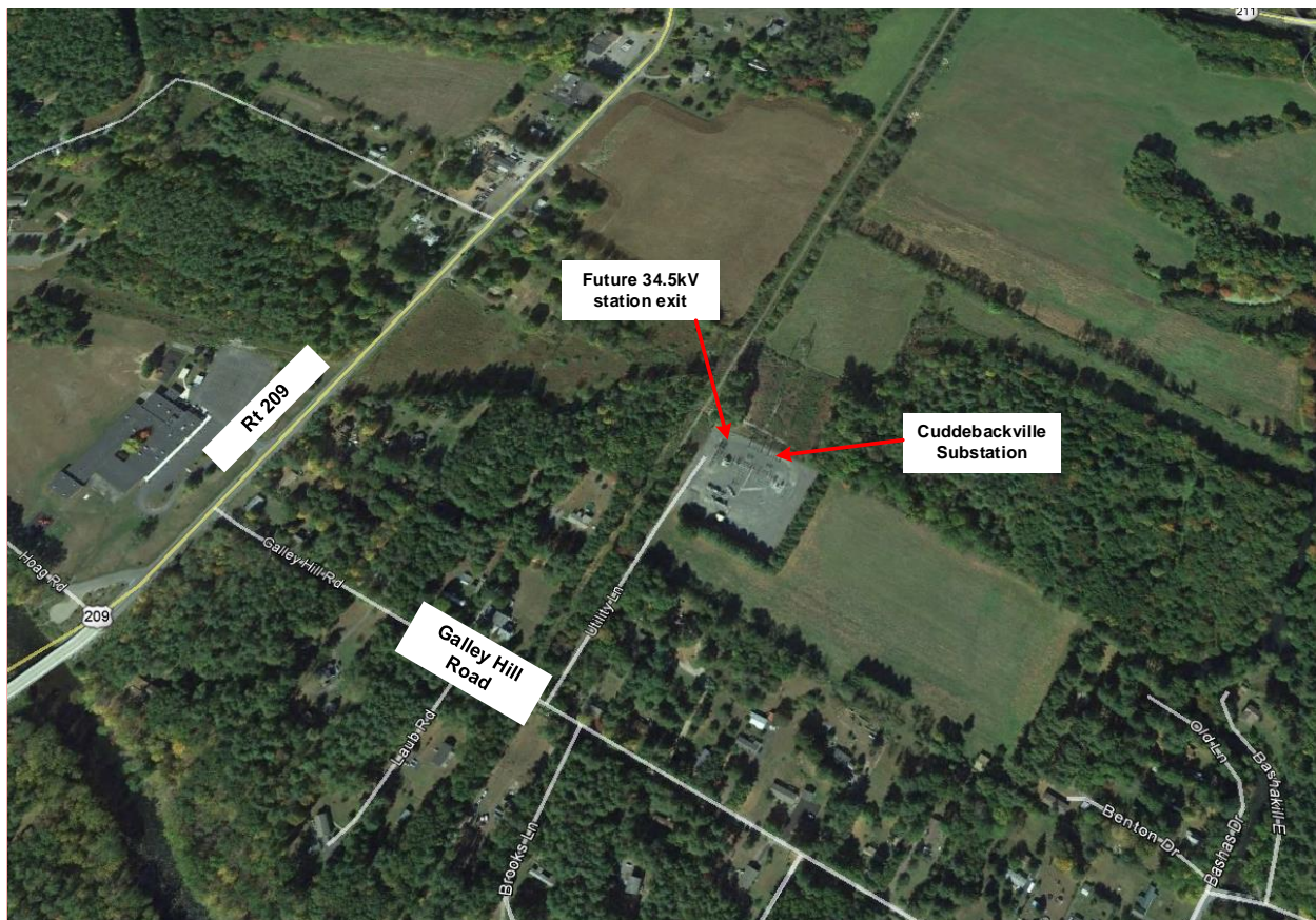
Address of the station: 49 Galley Hill Rd, Cuddebackville, NY
