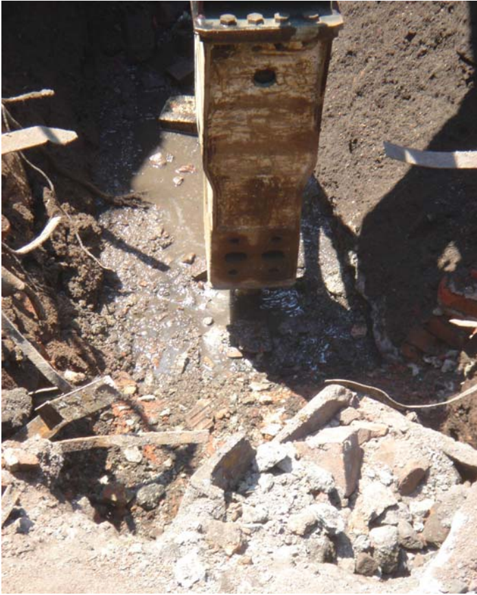
3. Hammer bit breaking the concrete slab at PBL-9.
