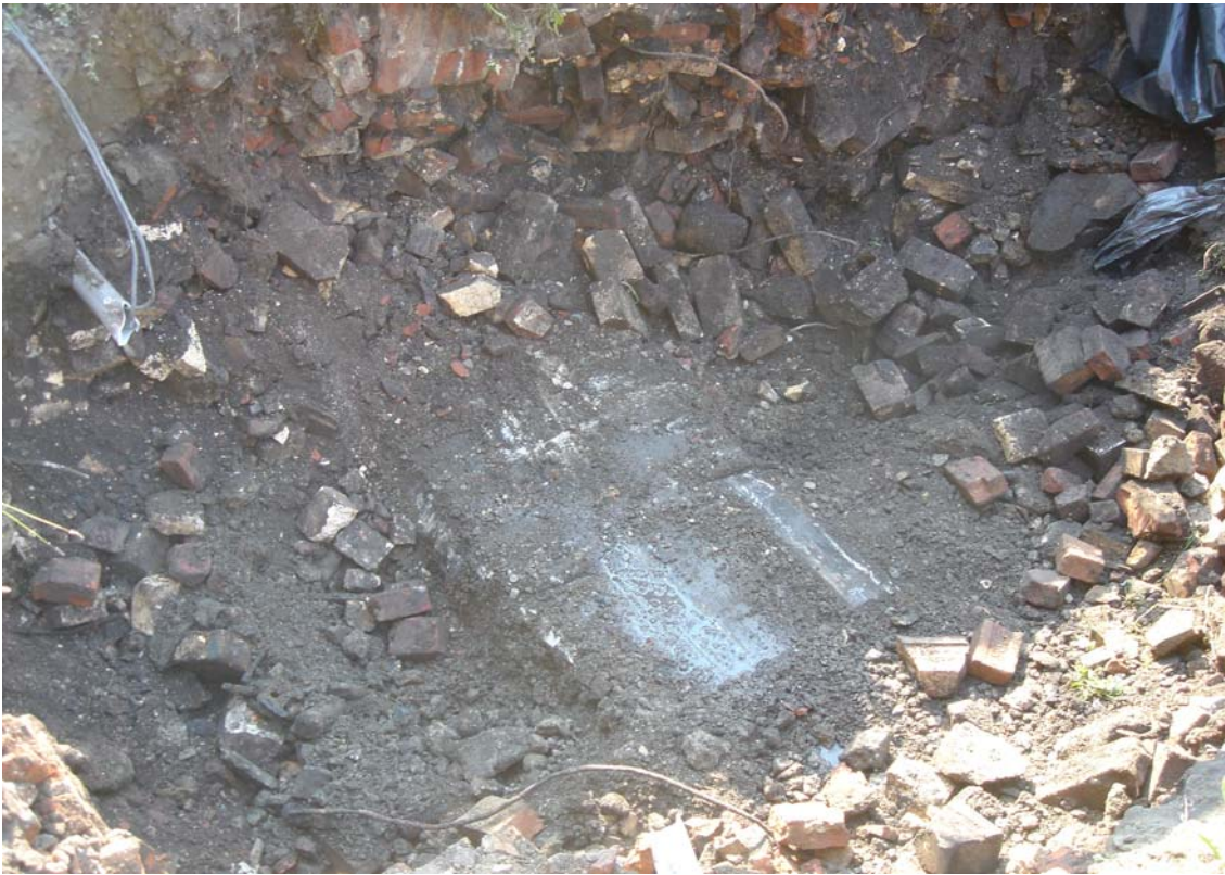
2. Test pit PBL-4, steel beams and concrete slab at 4.5 ft.
