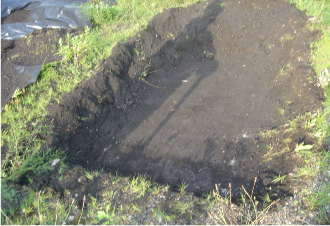
1. Test pit at PBL-1, concrete slab at a depth of 1 ft.
