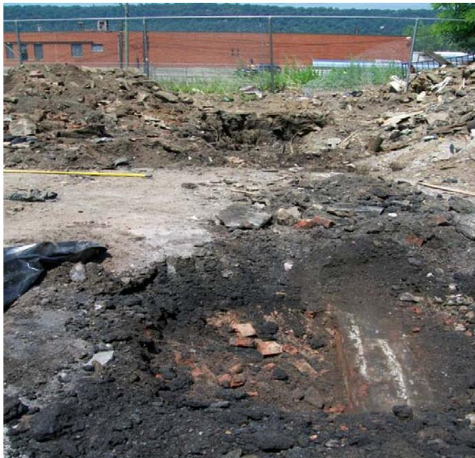
TP-2 eastward extension with exposed holder foundation wall and larger excavation in back ground
